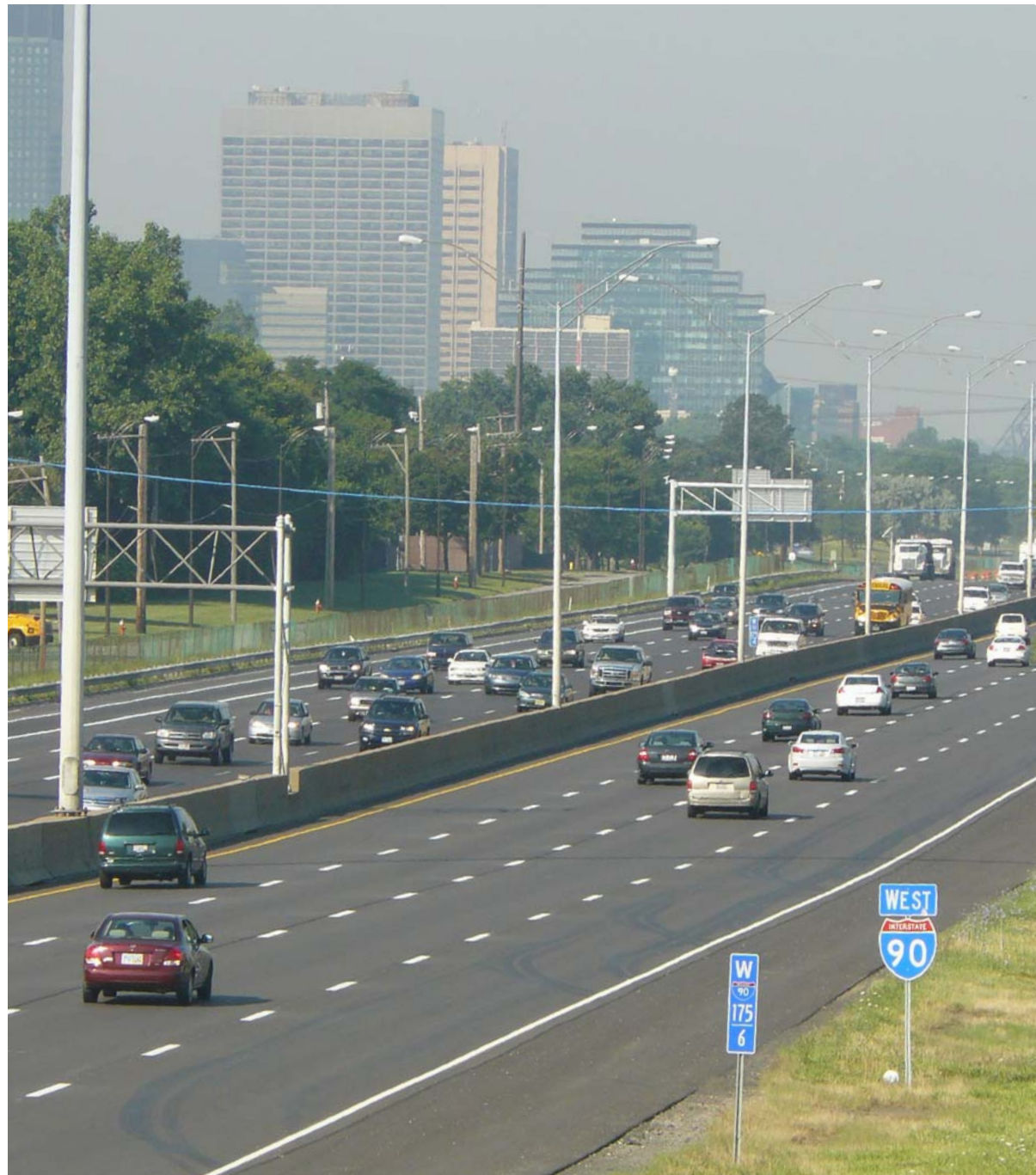
The East Shoreway looking west from East 55th Street – another successful Local 860 paving project
