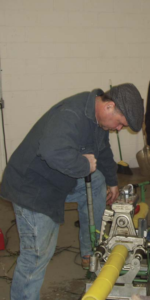
Ronald J. Skillicorn working on 3-inch pipe fusion
