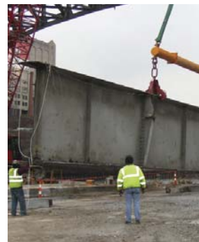
Widening girder on I-90
