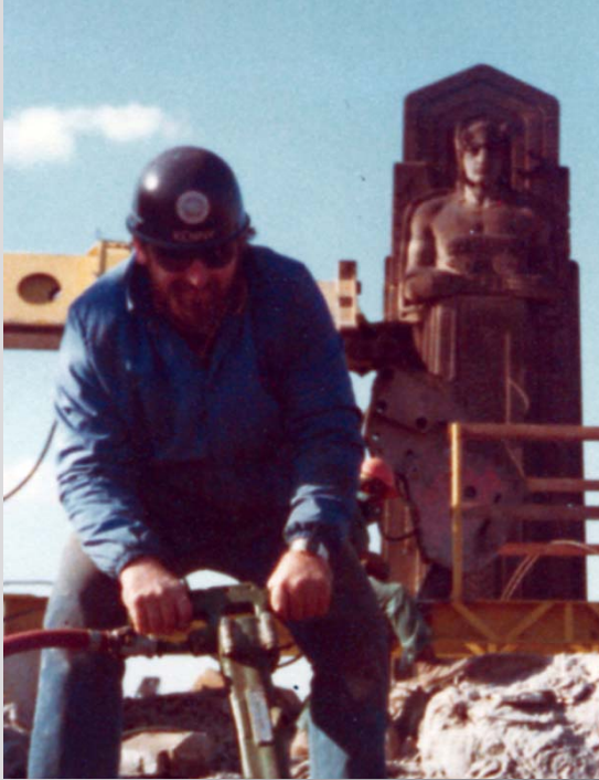
Kenny Yuko working on the Lorain-Carnegie Bridge.
