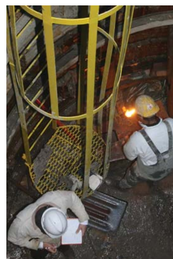
Building the shaft leading into the interceptor
