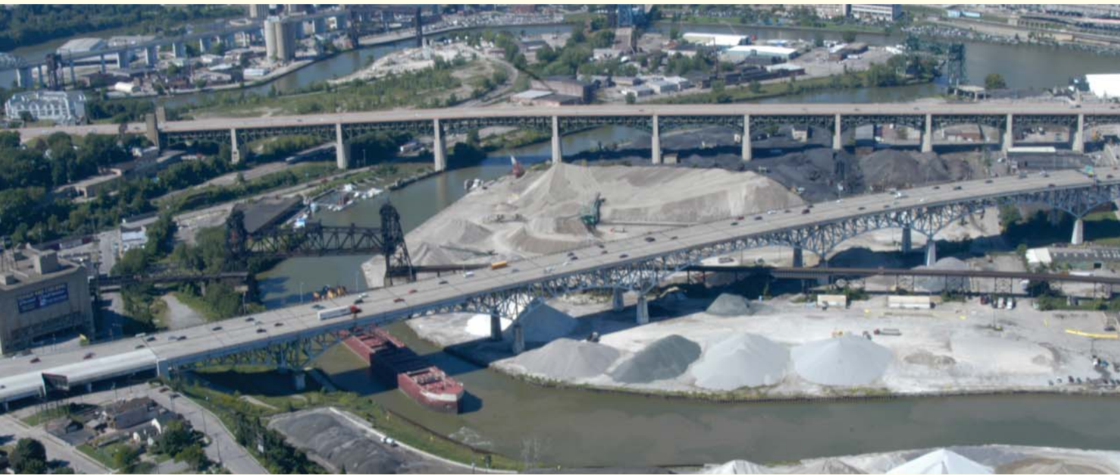
The Cleveland Innerbelt Bridge.
