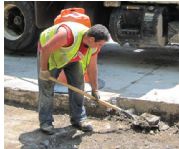
Below, on Pleasant Valley Road – John Paulica; Pleasant Valley Road resurfacing
