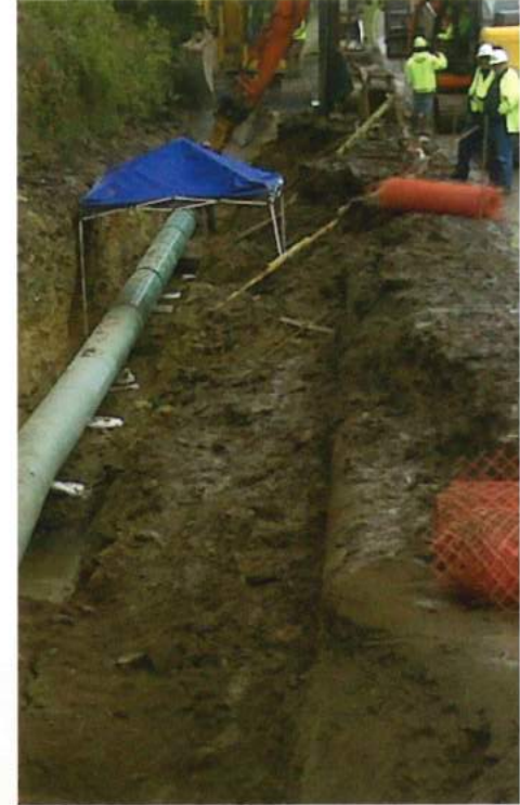
Pipeline work in Brecksville Photo courtesy of Dominion
