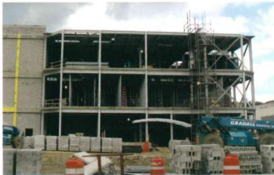
Southerly Wastewater Treatment Plant, Renewable Energy Facility, Kokosing Construction Co.
