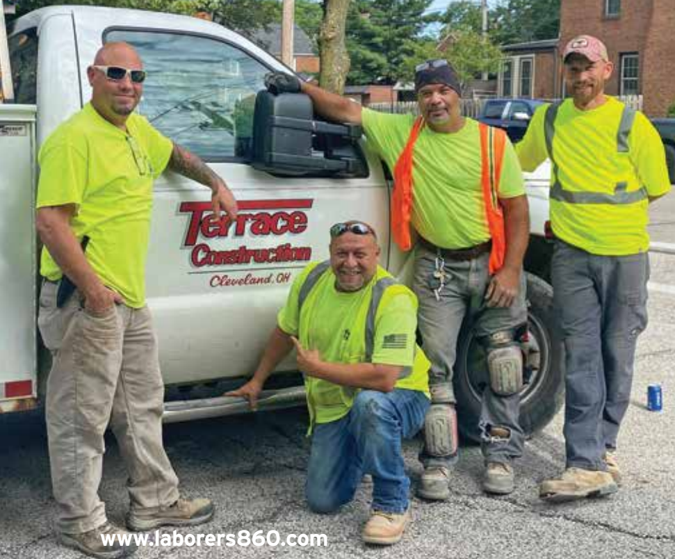
TERRACE CONSTRUCTION TRAYMORE WATERLINE PROJECT Lee Tarajcak, Billy Carmigiano, Orlando Santaella, Matt Lynn
